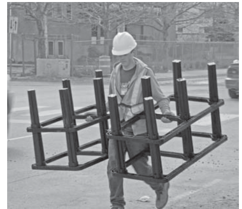
Silva Cells being moved to the trenches.
