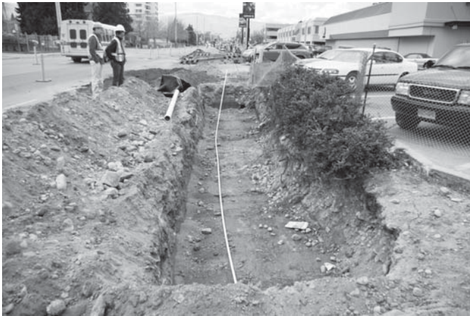
Excavated trench, ready for installation of soil cells.
