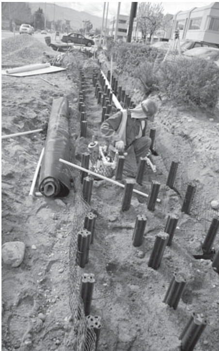
Assembly of soil cells and irrigation pipes.
