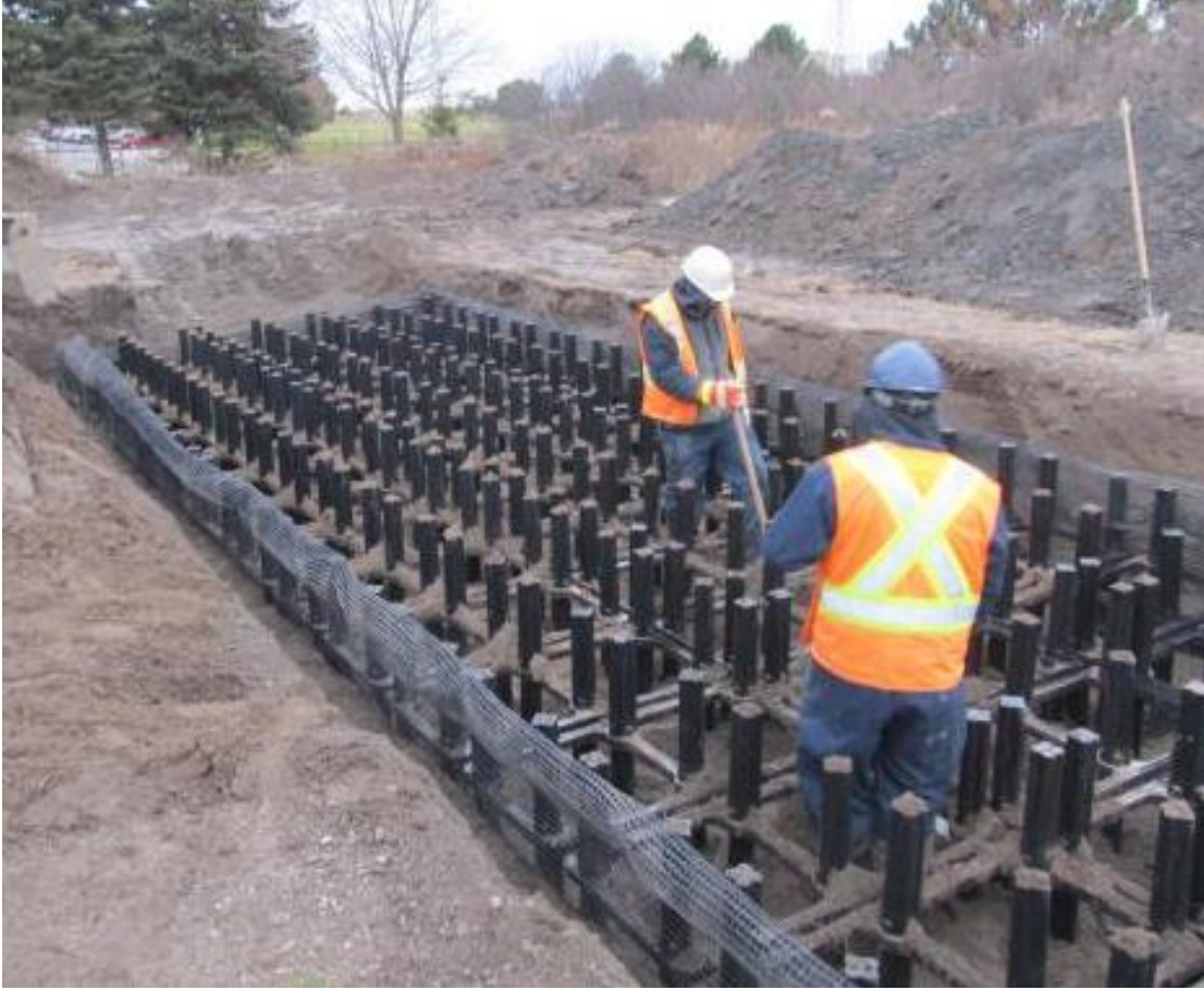
A typical Silva Cell system is constructed over the buried pipe
