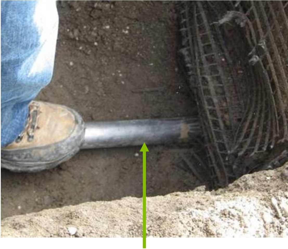
Boring head or Pneumatic -gopher going in on one side
