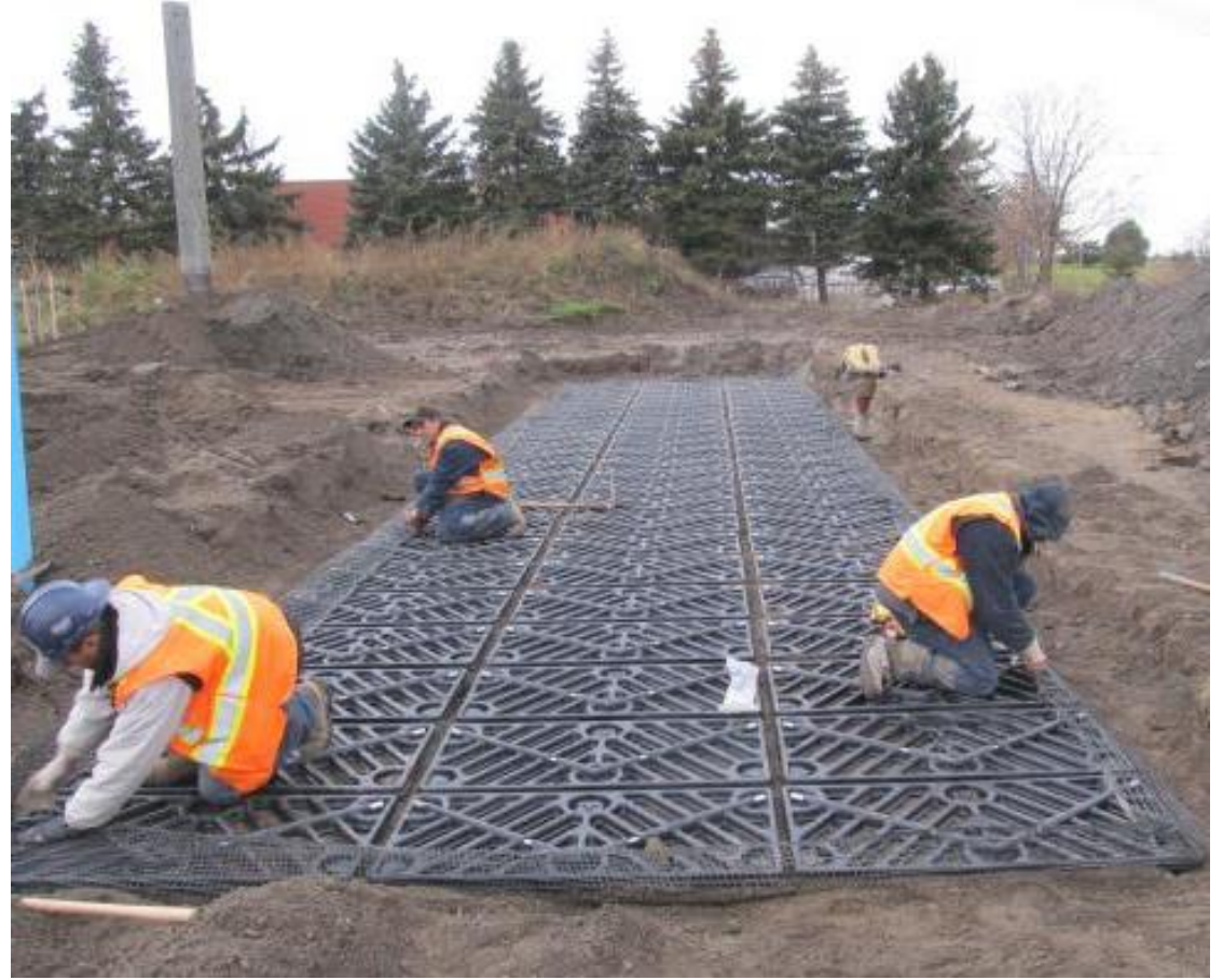
A typical Silva Cell system is constructed over the buried pipe
