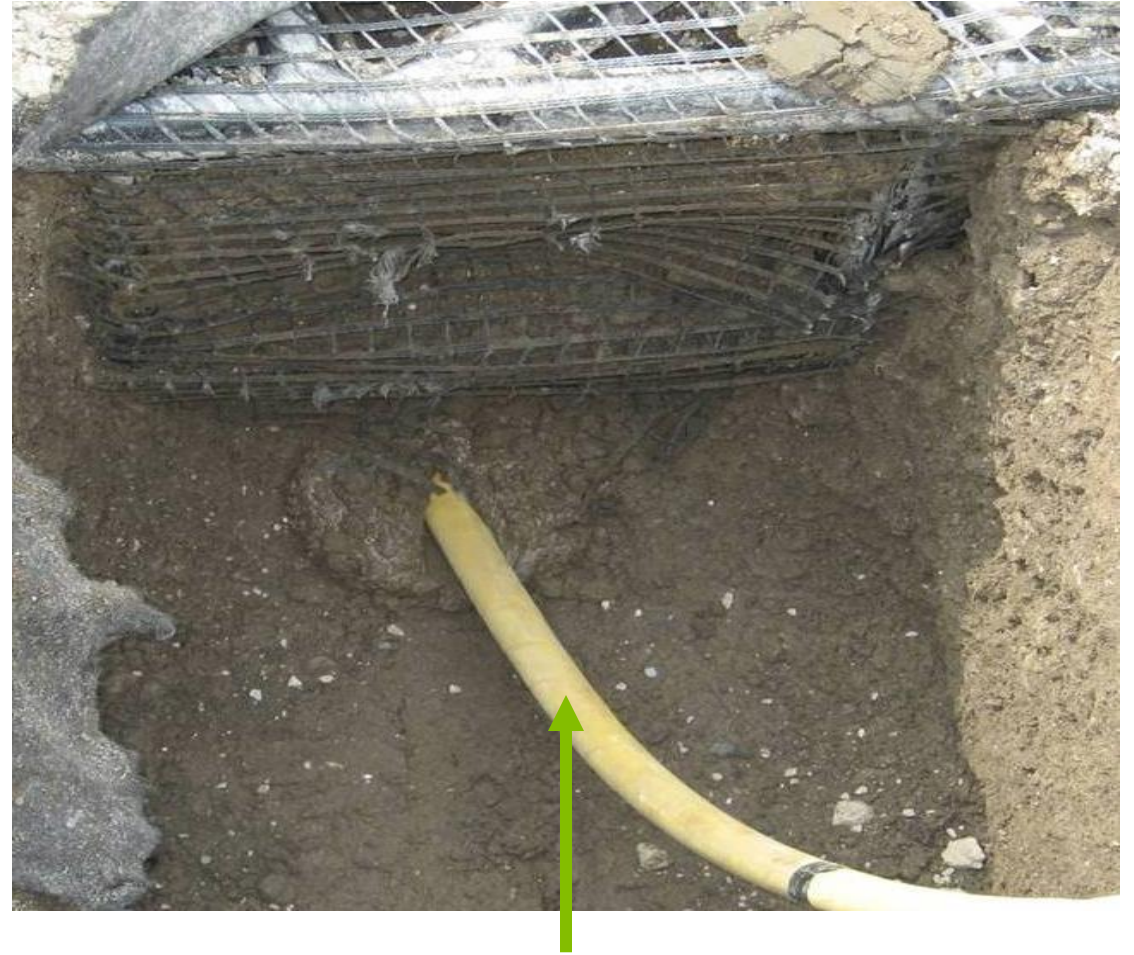
Boring head or Pneumatic-gopher coming out the other side
