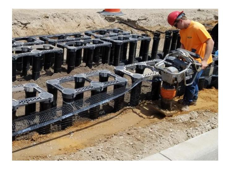
Keep compaction equipment from coming into direct contact with the legs to avoid potential damage.
