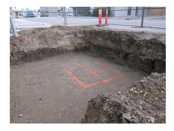
Mark out the inner dimensions of the tree opening
