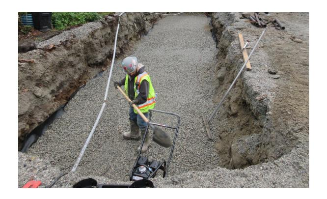
Fine grade the subbase aggregate to a uniform elevation or slope.
