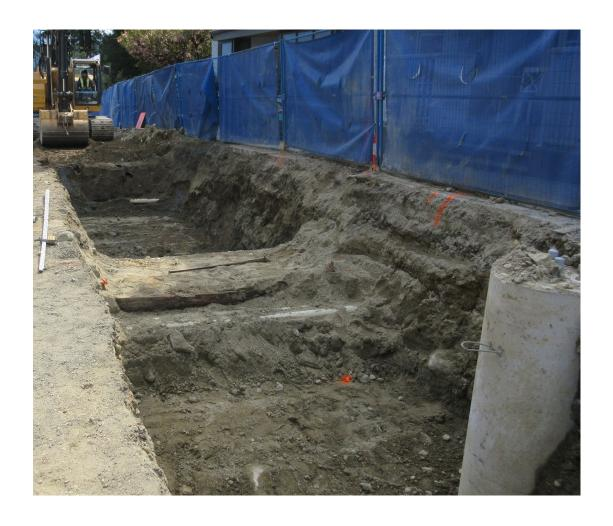
Make sure excavation is deep enough to accommodate subbase aggregate + Silva Cells + pavement section
