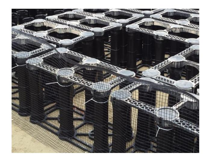
Attach geogrid with a cable tie at the top of each post to keep geogrid in place during backfilling
