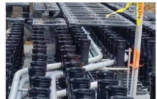
The Silva Cell provides the utmost in project flexibility, able to integrate utilities throughout the system.
