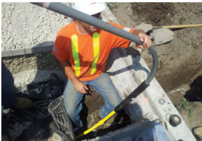
Riser is attached and pulled through.
