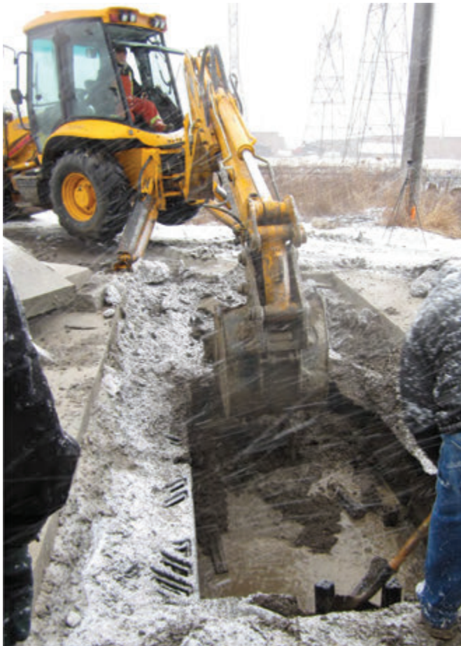
Mechanical removal of soil cells.
