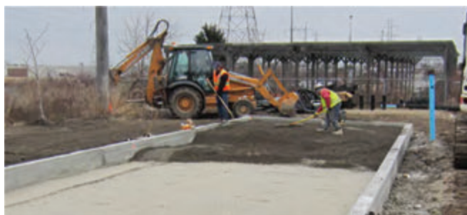
Backfill installation on top of deck.
