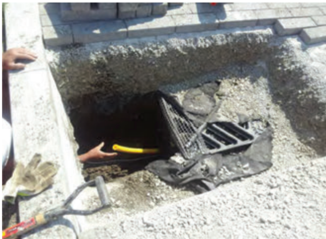
End of lateral at building end.
