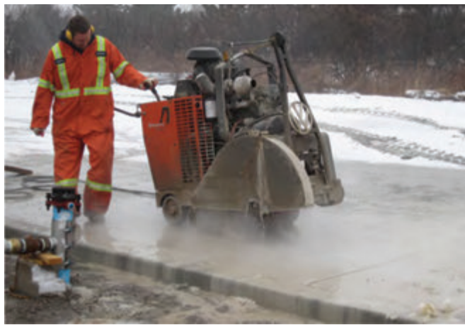
Sawcutting concrete pavement.
