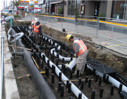
Perforated distribution pipes are placed throughout the system
