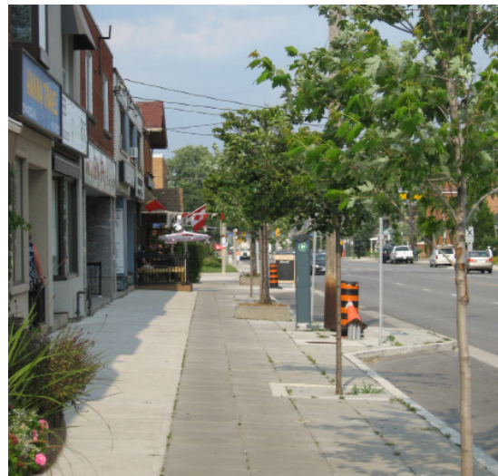
Asphalt covers the parking bay and pavers cover the sidewalk.
