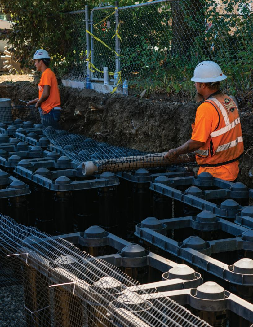
recommended. This is a minor additional expense and provides a means to drain the system if infiltration rates are lower than expected. The underdrain can be uncapped to convert the system to a filtration system.
