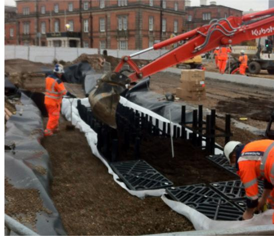
to be added in order to prevent settlement and act as a separator between the soil and clean angular stone backfill.
