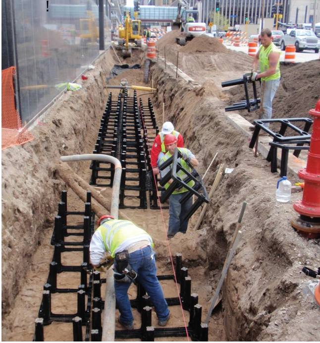
Above: Images of trees installed with Silva Cells and Pervious Pavers in combination with concrete sidewalk in downtown Minneapolis, MN, streetscape
