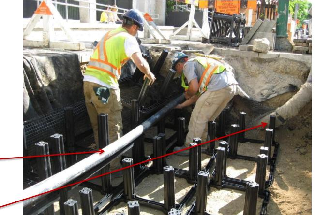
The Silva Cell frames are filled with soil , the decks are attached and the geotextile fabric is patched
