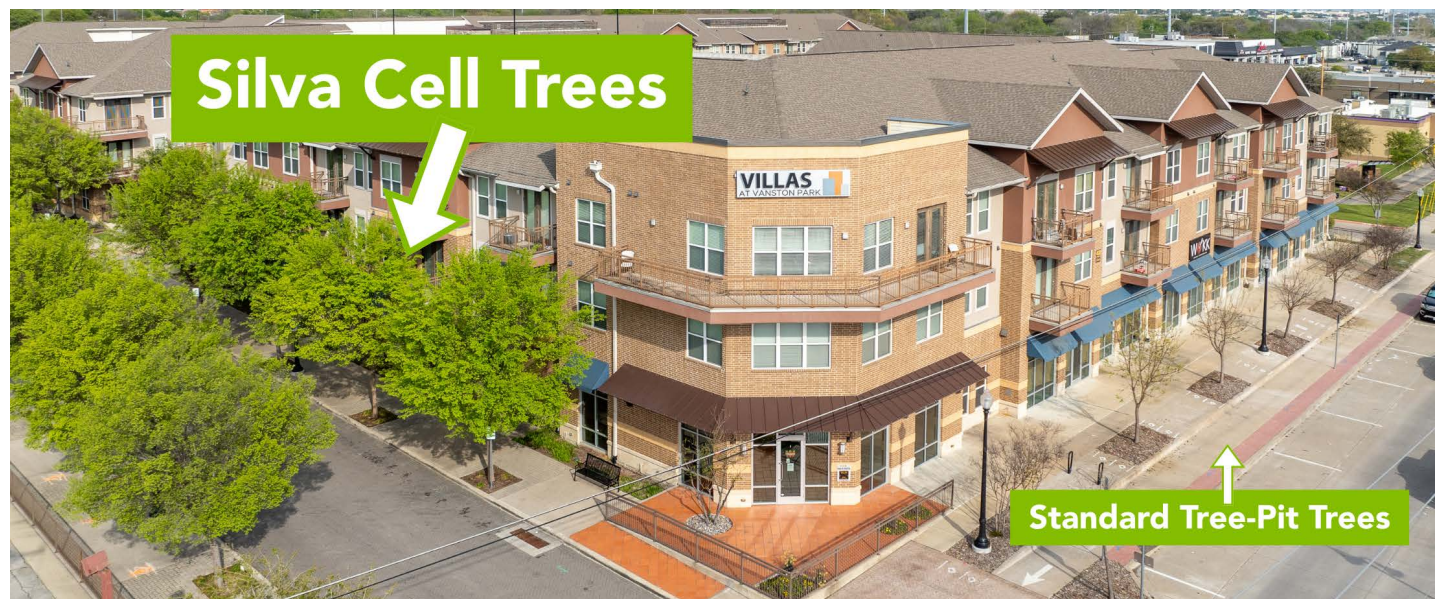
Silva Cell trees (left, Lacebark Elm, 8 years of growth) versus traditional pit trees (right, Chinese Pistache, 5 years of growth). Silva Cell soil volume is approximately 500 ft 3 per tree. Mesquite, Texas, 2024.
