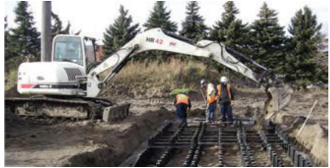
Soil cell trench filled with soil.
