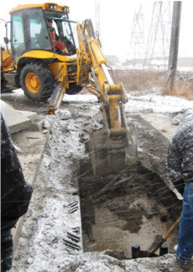
Mechanical removal of soil cells.
