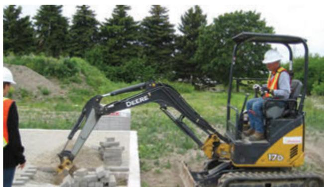
Removal of pavers and granular base.
