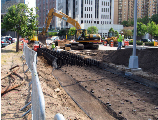
A bioinfiltration soil mix is used to fill the system.
