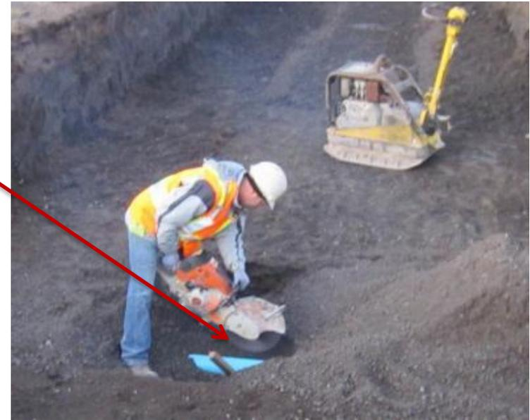
**A saw cut was made into the pipe to act like a break in the pipe**
