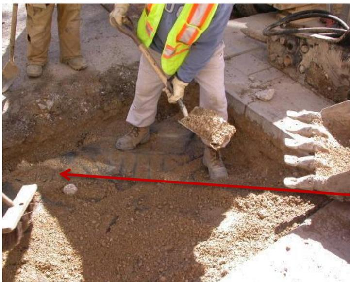
**The aggregate base is removed and the fabric covering the decks is cut and removed**
