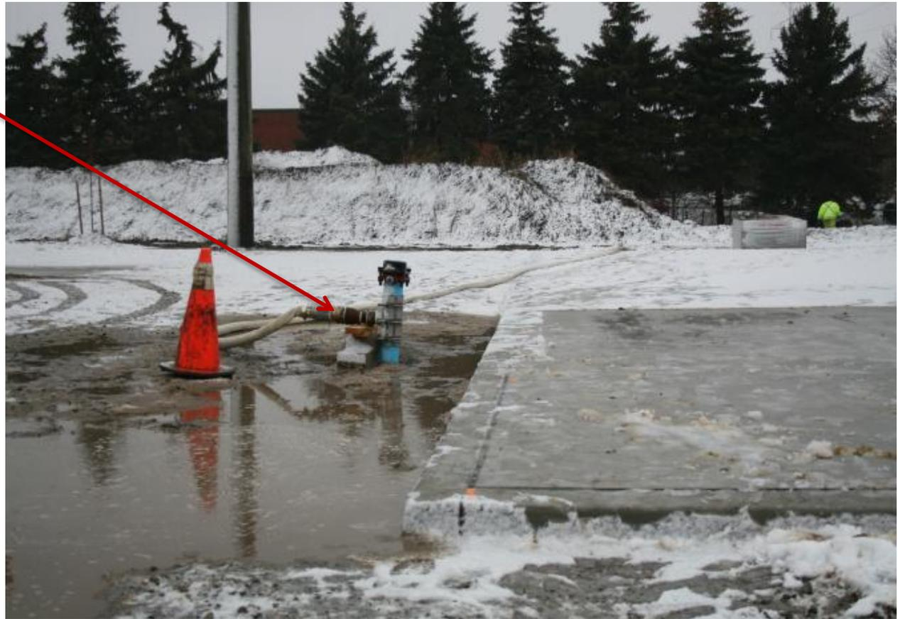
\*Due to the soil in the Silva Cells being loosely compacted, the water came to the surface very near to the location of the break rather than traveling underground
