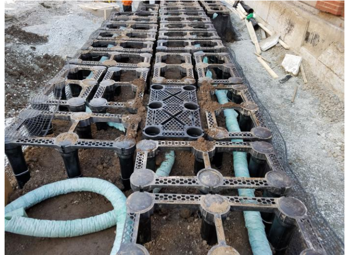
Distribution pipe shown within ponding depth
