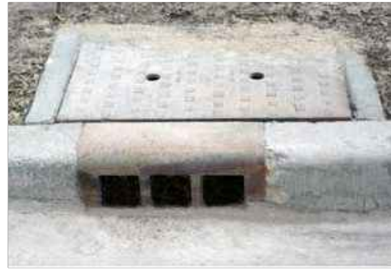
1 STORMWATER TREE APPLICATION | STORM.xCC1 | SAMPLE INLET IMAGE CC1-2 NOT TO SCALE
