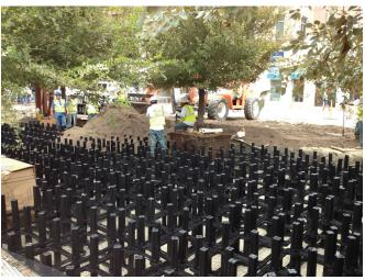
amended soil panel below due to large crowds during events. Grading in the plaza was designed to slowly sheet water into the allée, and decomposed granite was used to prevent runoff. Water efficient irrigation techniques were used in the allée to help sustain the trees during the hot Texas Summer months."
