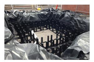
derdrain was also installed, resting inside the Silva Cell structure on the frame at base. A 350 m<sup>2</sup> thrust block/ concrete surround was cast in place around the standpipe connection to the underdrain.
