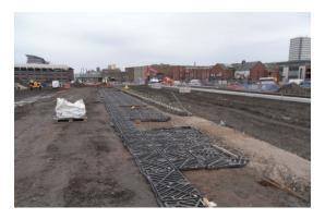
And it is indeed a large scale: altogether, 1,772 frames and 866 decks were installed in a two layer system along the boulevard, bringing 16.18<sup>3</sup> of soil volume to each of the 31 newly planted trees. Through this ambitious creation of a new, tree-lined pedestrian-friendly passageway, Sunderland's vision of a vibrant and prosperous city centre is one tremendous step closer to realization.
