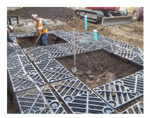
The resulting system allows all of the runoff for the plaza to go directly into the soil contained in the Silva Cells. Underdrains provide a route for excess water to run off if necessary. Since all the stormwater from this part of the campus flows in to nearby Strawberry Creek, the University was concerned about controlling the quality of the runoff. By filtering all the plaza runoff through soil stored in the Silva Cells, they are able to maintain this quality control on-site.
