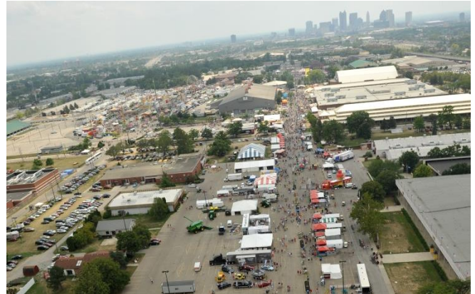
The fairgrounds prior to 2013 did not have adequate shade, and the lack of shade was not inviting to visitors. The installation was completed in April 2013.
