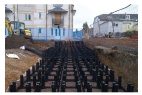
were planted in a strip of land near the corner of the building. Stormwater enters into the Silva Cell system through the lawn surface and permeable surface of the car park. In total, 198 Silva Cell frames and 99 Silva Cell decks were installed in a two layer system alongside the car park, bringing each tree 18.7 cubic meters (660 cubic feet) of soil.
