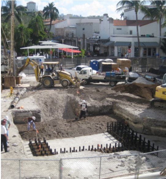
The installation around the water gardens begins.
