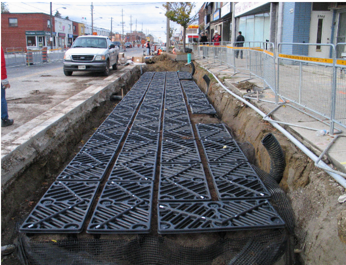
Silva Cell decks go on
