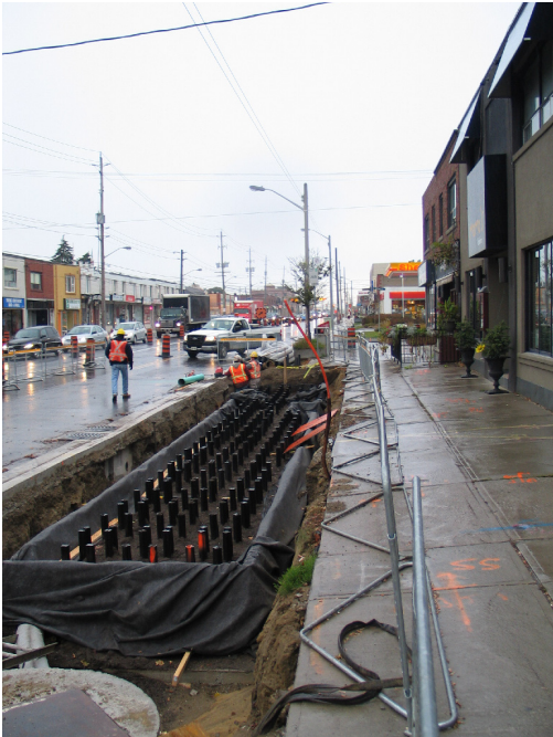
Silva Cells are laid out
