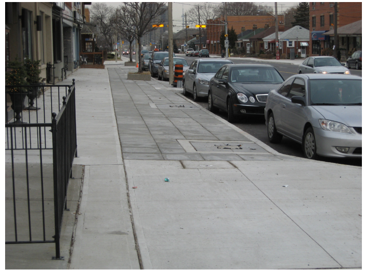
Asphalt covers the parking bay and pavers cover the sidewalk. Two new trees will be planted in the Silva Cell trench in Spring 2009.
