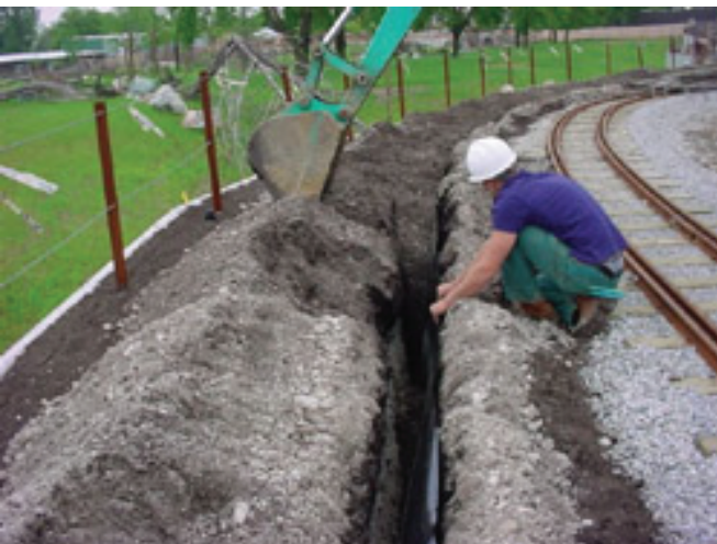
Installation of BambooBarrier™
