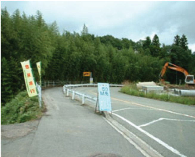
Damaged Multi-Use path
